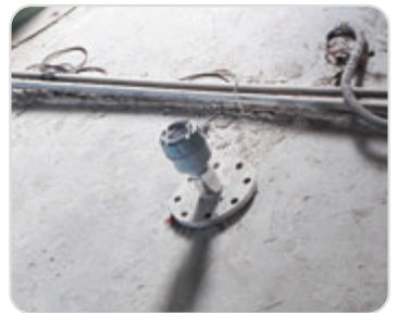
Feeding plant Corn storage tank detection
