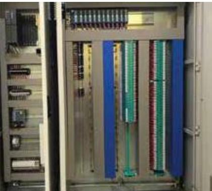
The PLC stands for Programmable Logic Controller and SCADA stands for Systems Control and Data Acquisition. PLC panels are a type of control panel that is programmable to the required sequence and also follow the flow of the process. A powerful CPU acts as the main brain for controlling all the other panels and machines. PLC Panel designed for controlling various manufacturing processes and ideal solution for automation.
