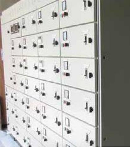
MCC stands for a motor control centre, MCC Control Panel consists of feeder for motor and blower and designed especially for motor operations. The MCC receives a signal from the control panel and which is used to control motor. The MCC is directly connected to the analogue motor. They are most commonly used in industrial and commercial facilities where there are plenty of electrical motors at use.
